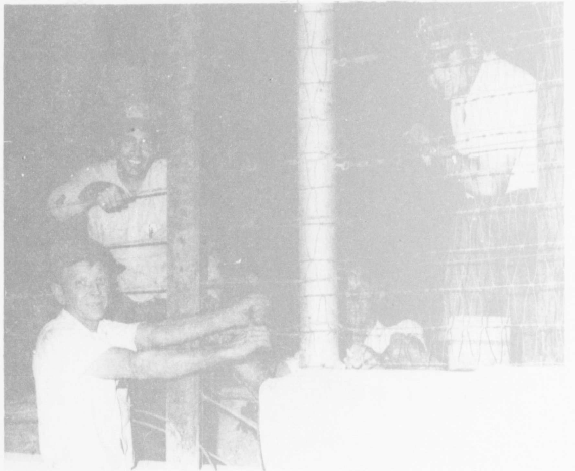
This year the Jaycees have constructed a concrete wall on the west side of the arena. The wall (over 240' in length) required over $1000, in materials and over 500 night man hours of labor (no charge). Just part of the work crew are pictured above (left to right) Cotton Warren, Bill Henson, Dee Burt (almost hidden by steel post) and Jack Poston (behind wire).
