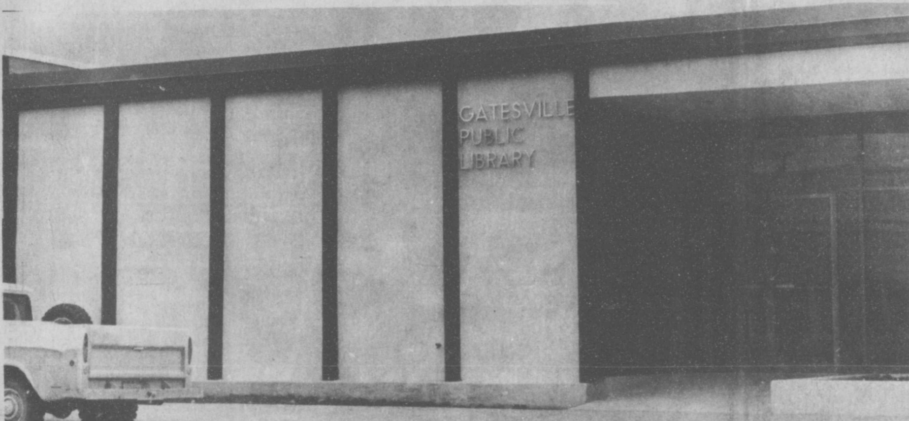
Texas State Library representatives, city officials, library board members, and Friends of the Library gave final approval of the new modern Gatesville Public Library building Wednesday afternoon. The officials tour occurred just three days prior to Na-
