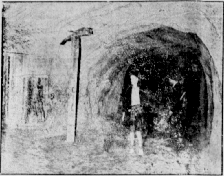
The mile-long tunnel under the Palos Verdes, dug years ago as a mine, can withstand a great deal of shock, has twin entrances, a lighted branch tunnel, and a number of vents. Joan Fargo, 15, and Edsel Newton, of Watteria, Calif., test it as an air raid shelter.
