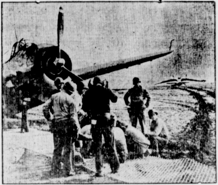
METAL MATS FOR DESERT TAKEOFF—When Anglo-American forces occupied North Africa, torpedo planes took off in the desert on metal mats like this one, which formed temporary airfields.
