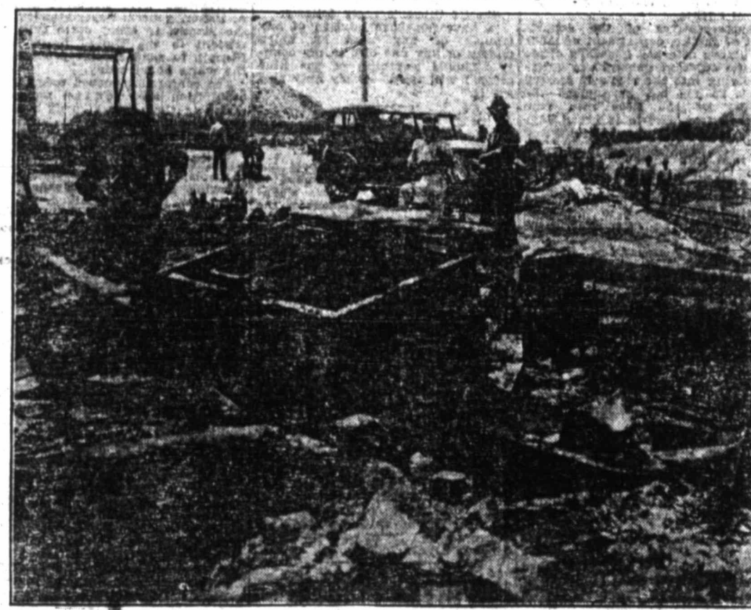
Above is what was left of the demolished offices of the Southern Illinois Coal Company, at the mine. After the fighting ceased the large safe shown in the foreground and said to have contained considerable money, was opened by dynamite and the office building burned to its foundations.
