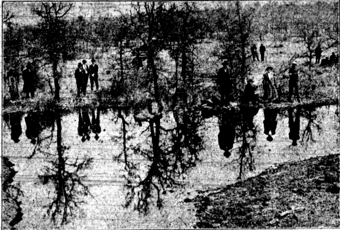
Above is shown earthen storage tank which could tank improvised by damming up a hole and pipe line connected to rough hollow to take care of producing the new Gulf Production Company's No. 1 Hookaday, four miles south of Graham which was flowing Saturday at the rate of 2,000 barrels per day.
