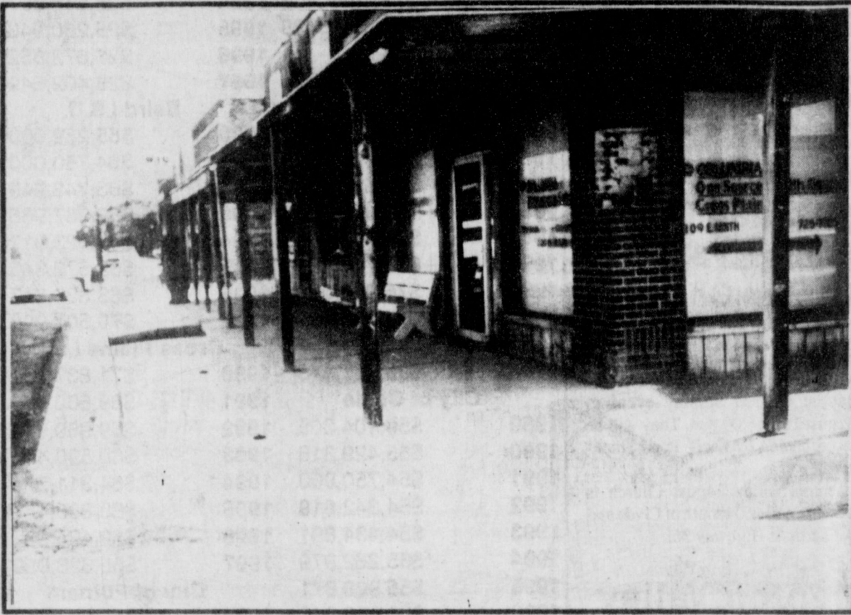
SIDEWALK PHASE I COMPLETE — A view of the corner of 9th Street and Main shows off the new sidewalks. Phase II will begin sometime after Homecoming.
