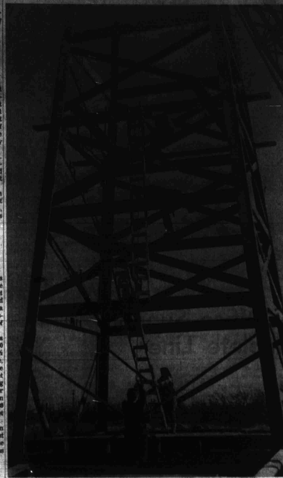
BUILDING A DERRICK — Employees of the Shorty Hall Rig Co. of Odessa prepare outside exhibit for the Permian Basin Petroleum Museum, Library and Hall of Fame. When completed, the derrick will be over the original drilling and producing equipment of Santa Rita No. 2, the second well in the Big Lake Field of Reagan County.
