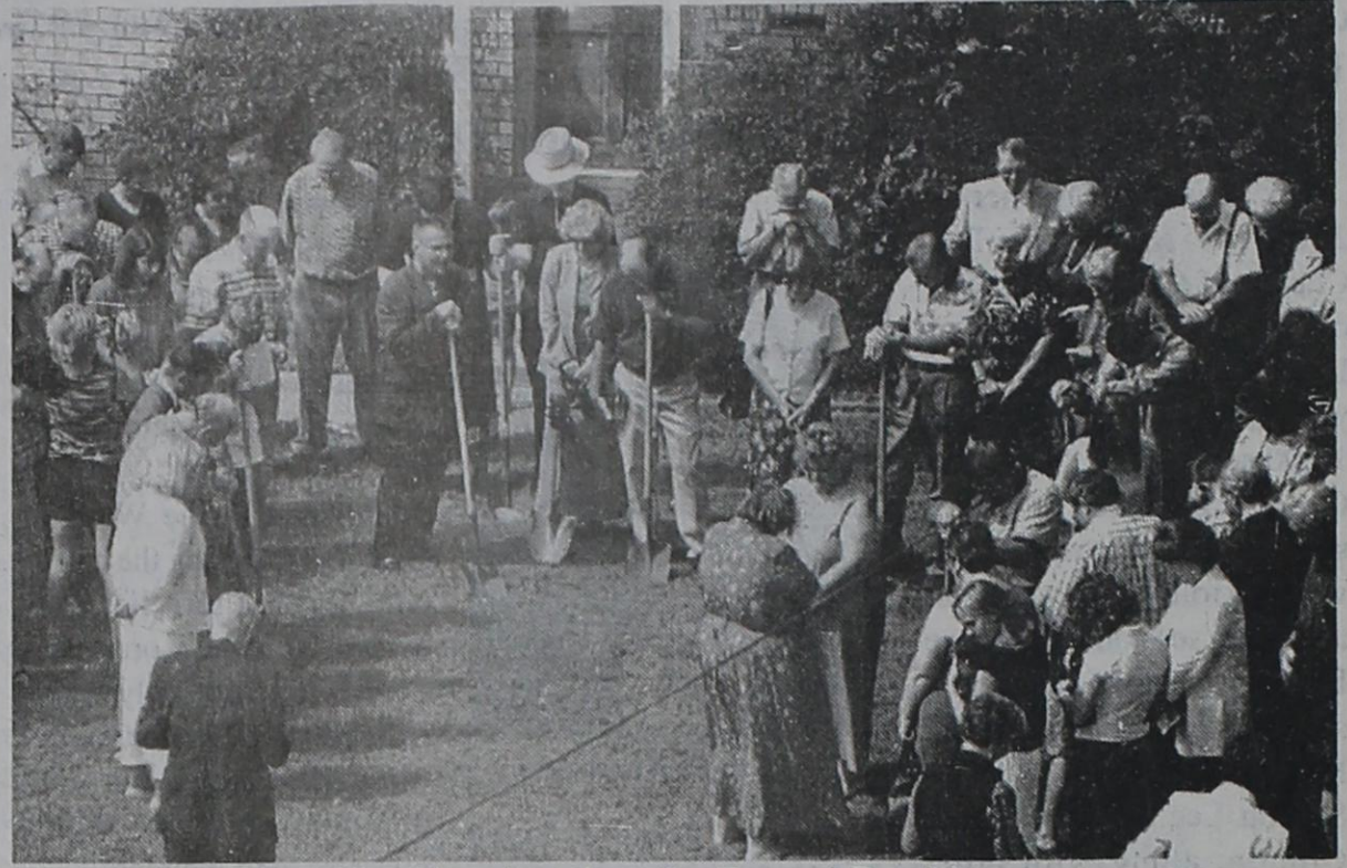
The Church gathers for Ground Breaking.
