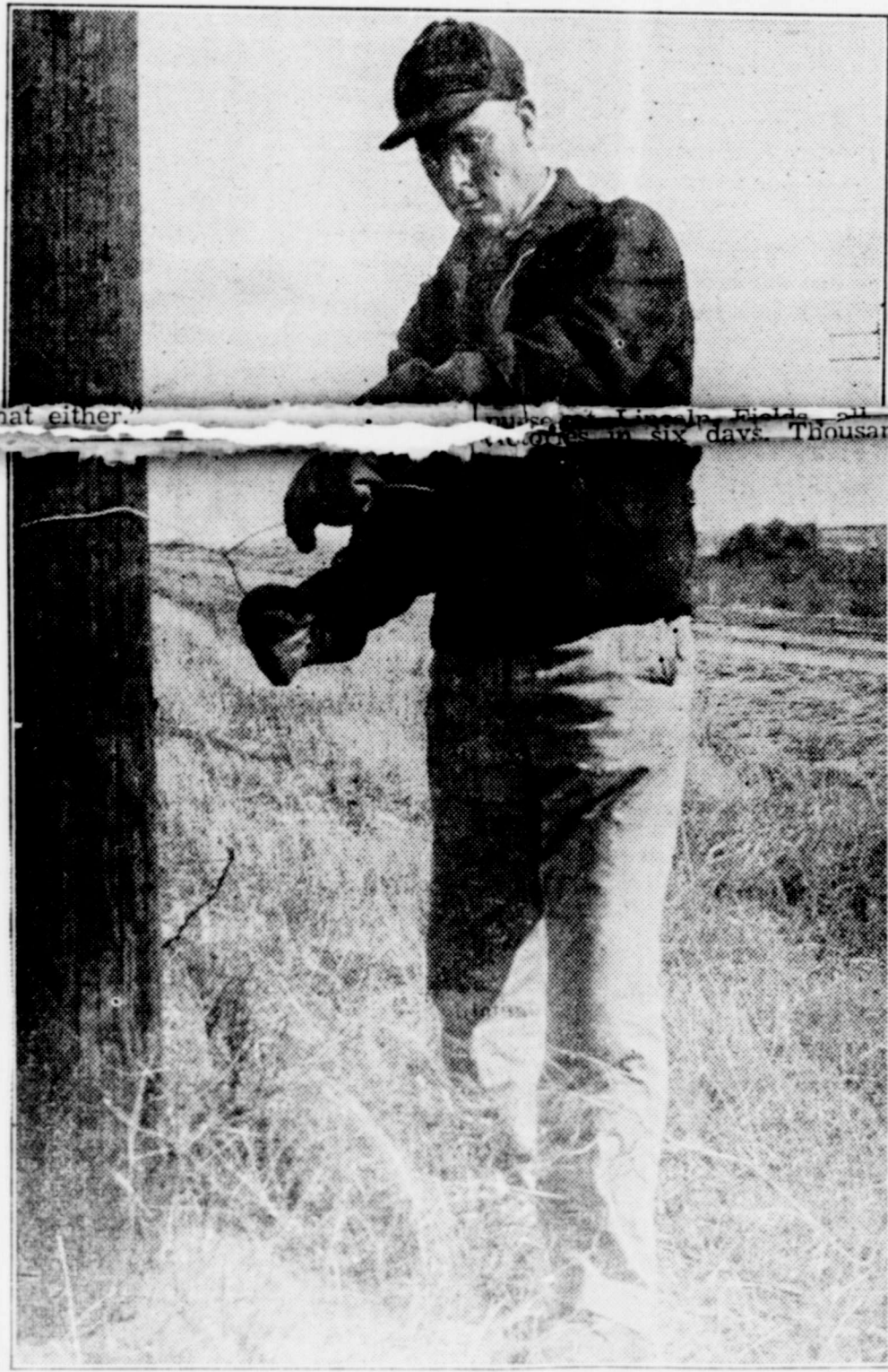
Lineman J. B. Handley of Childress shows how ordinary fence wire was used for climbing hooks in emergency that won national honors.
