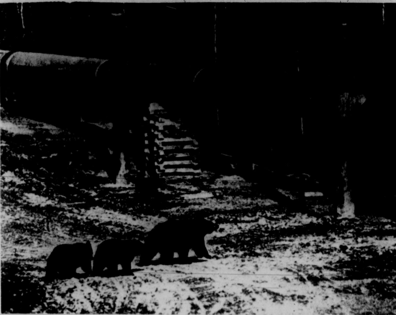
A BEAR AND her cubs meander across the trans-Alaska oil pipeline right of way, passing under an elevated section of the 800-mile-long line. The elevated sections were among the demands won by environmentalists who battled the original engineering design. Environmentalists said a ground level line could block normal migration movement.
