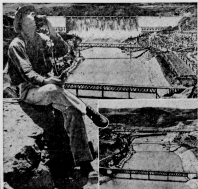
While supervisors guide concrete buckets by telephone, Grand Coulee takes shape. Upper picture shows how it will look when finished, compared with lower photo showing present status.
