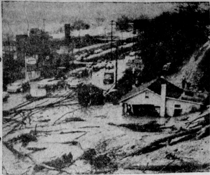
LANDSLIDE BLOCKS U. S. HIGHWAY — A landslide blocking U. S. Highway 52 in Ohio, across the Ohio River from Ashland, Ky., reached a depth of about eight feet in yellow mud, tree branches and limbs and other debris. Shown above, a service station office owned by W. R. Newman of Ironton, Ohio, is being collapsed by the force of the creeping mud. The slow-moving landslide threatened to close the main line of the Norfolk & Western Railroad but a power shovel was moving the muck as rapidly as possible and the lines remained open.
