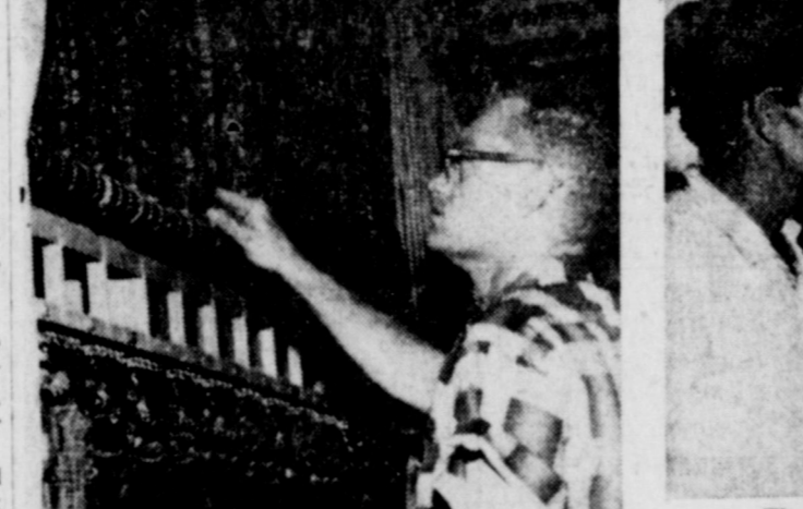
The picture above shows George Chapman at the main distributing frame where the 200 additional lines are connected to underground cable. This is where the lines go out of the central office building and eventually connect with our outside distribution cables.
