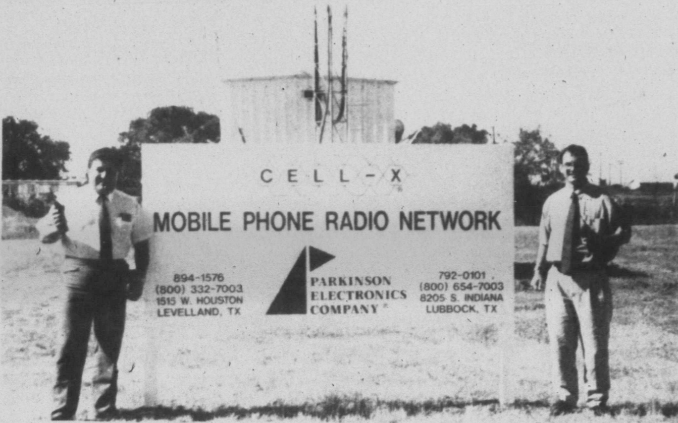
TOWER RELOCATED —Parkinson Electronics, headquartered in Levelland, recently erected a tower in Tahoka at S. 5th and Ave. M to allow local access through their Cell-X mobile telephone system to New Home as well as to Tahoka and Wilson. Previously the Cell-X equipment was located on the radi station tower west of Tahoka, and New Home calls were long distance. Those calls now are local through the mobile phone setup, according to Ron Davis, right, who is the Tahoka local representative, and Sammy DeLara, left, sales manager for the company. Behind the sign can be seen the lower portion of the tower, which goes up almost 200 feet.
