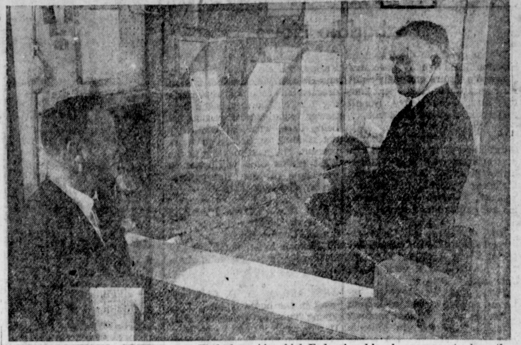
COMMUNICATIONS CENTER at Wadesboro, N. C., combines a round-the-clock civil defense nerve center with a unified radio service for local police, fire and sheriff's departments. Used for this dual purpose, the equipment is kept in top-notch condition at all times to meet emergencies. At the radio is Waldo J. Stroud, one of three operators hired by the local CD unit under a program in which Federal and local governments share the costs of new civil defense employees. Raymond H. Northcutt (right), Wadesboro-Anson County CD director, explains his radio setup to Herman J. Sisk, Area E director for the North Carolina Civil Defense Agency and one of five area directors hired under the same cost-sharing law to help build up CD at the local level. (OCDM Photo)
