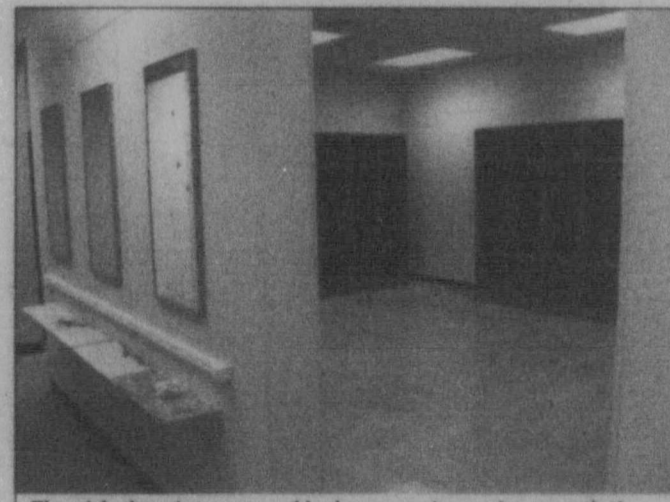
The girls dressing area and locker room is nearing completion
