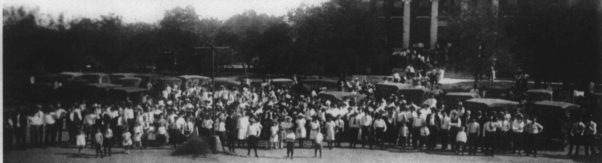
1920 Celebration ... A large crowd of citizens is shown in front of the nearly-new Lynn County Courthouse, before streets were paved, about 1920. This photo is on display at the Tahoka Pioneer Museum.
