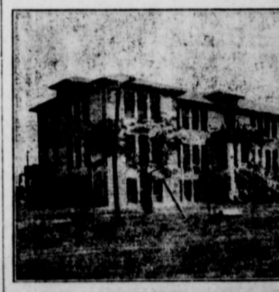
Pearsall's recently built high school building.
