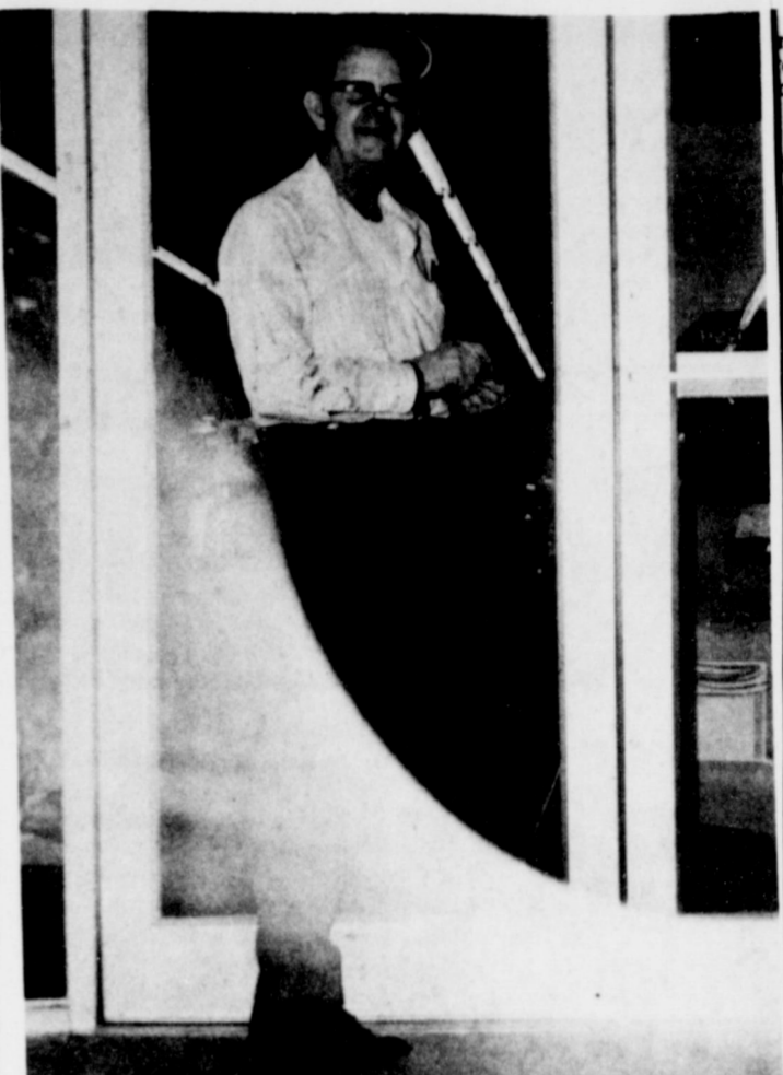
REPAIRING DAMAGED DOOR--Olan Burrows of St. Clair's was busy Sunday morning making temporary repairs to a glass door which was broken out Saturday night or early Sunday morning. This was one of the places with extensive glass breakage during the weekend.
