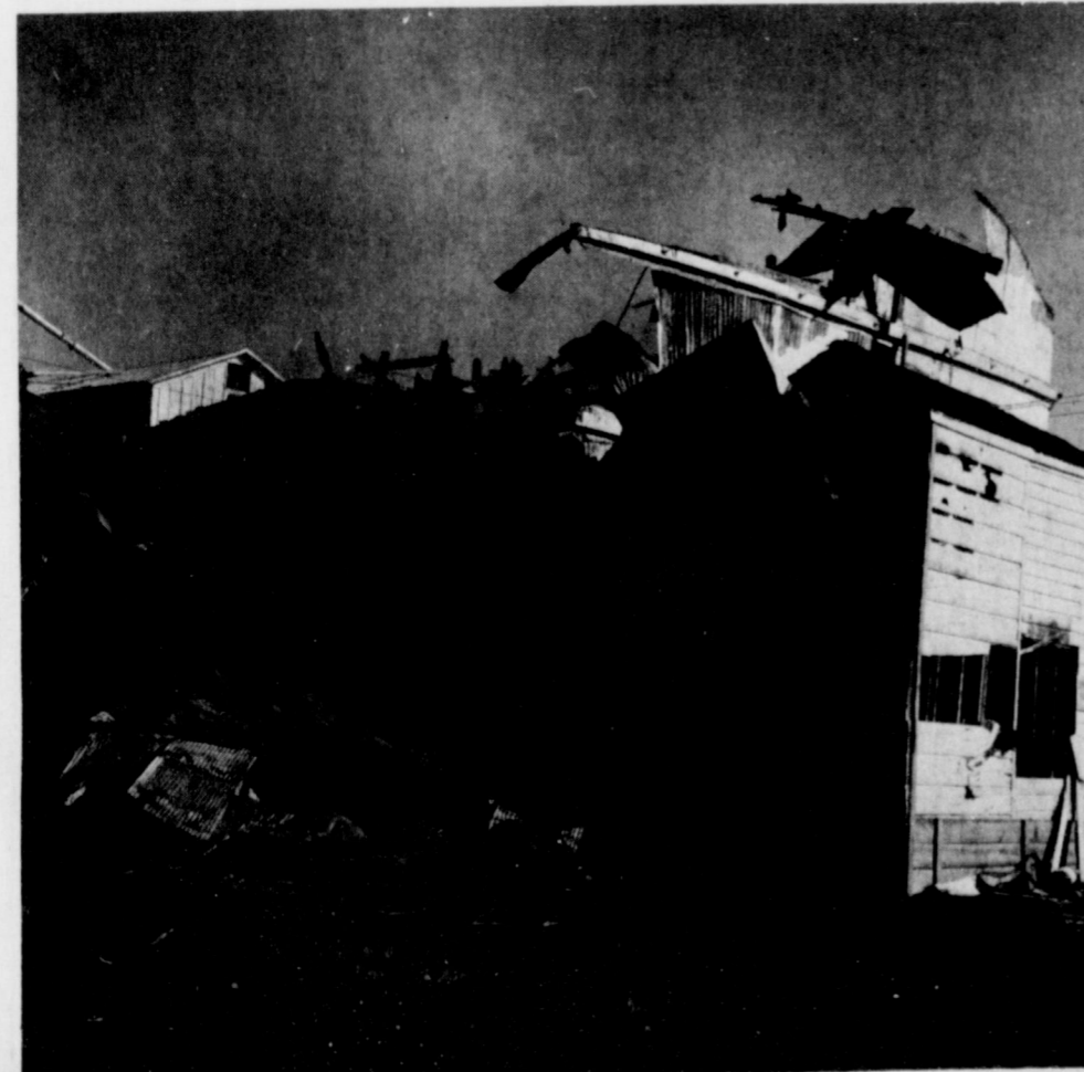
FIRE DESTROYS ELEVATOR AT FARWELL . . . The Kelly Green Seeds Company in Farwell was the scene of a devastating fire Monday night. Fire fighting equipment was sent to Farwell from Bovina, Friona, Texico, N.M., and the Clovis Fire Department who sent a special snorkel truck. Cause of the fire has not been determined as of presstime Wednesday.
