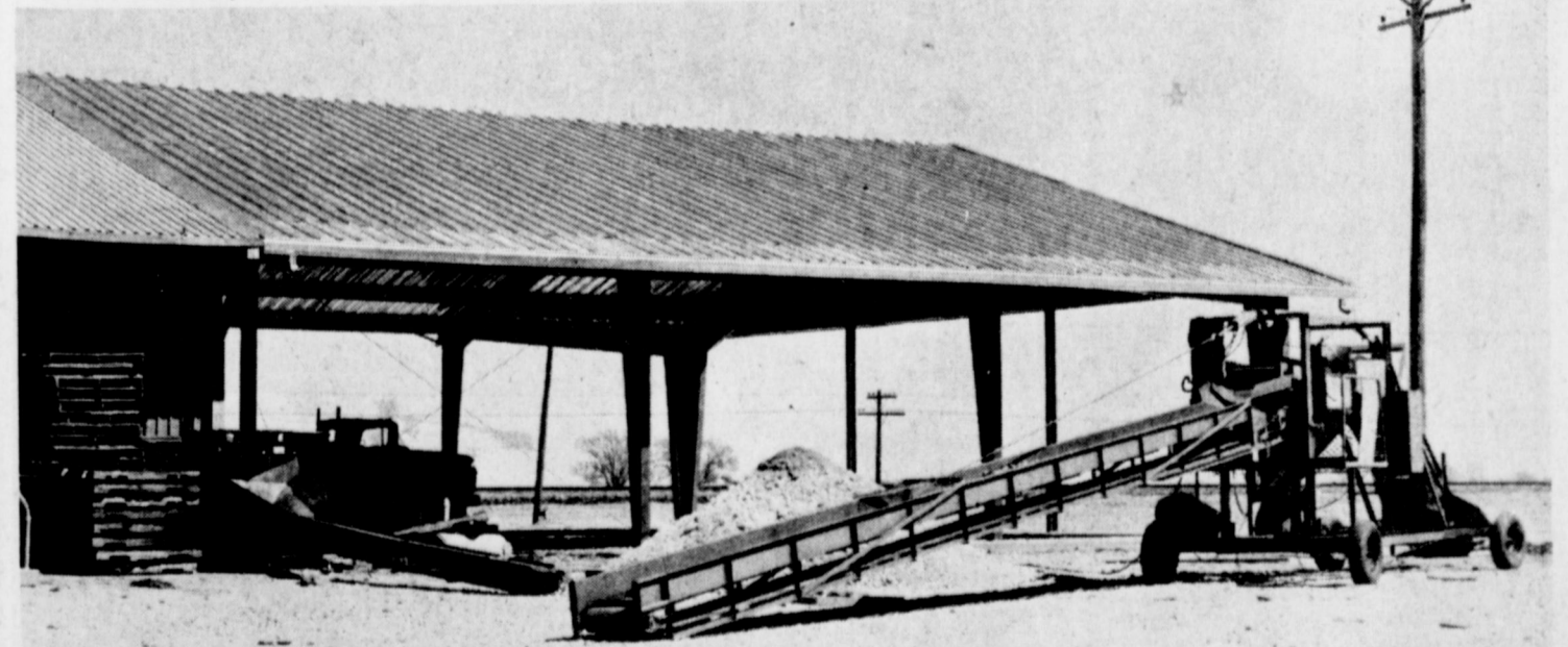
ADDITION MADE TO SHED . . . . . A building extension for storage and loading has been added to the T.J. Power Potato Shed in Muleshoe recently. Manager, Joe Tidwell, said that this year the firm has increased the acreage for potatoes in Bailey County by about 200 acres. This will make about 500 acres in the coun-
