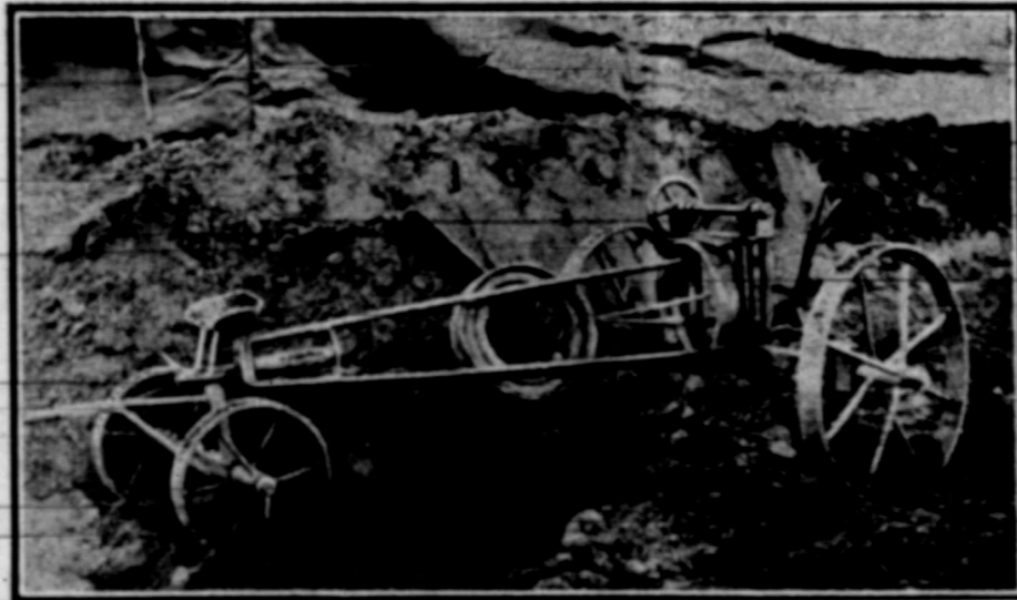
Showing the Grader Cutting Down Embankment on Roadside.
