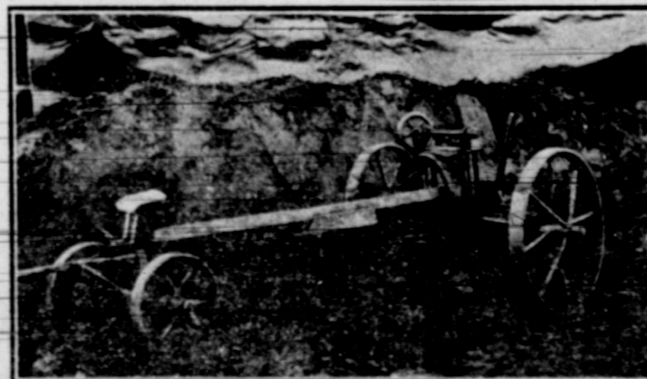
Moving Dirt to Proper Place After Cutting Down from Bank.
