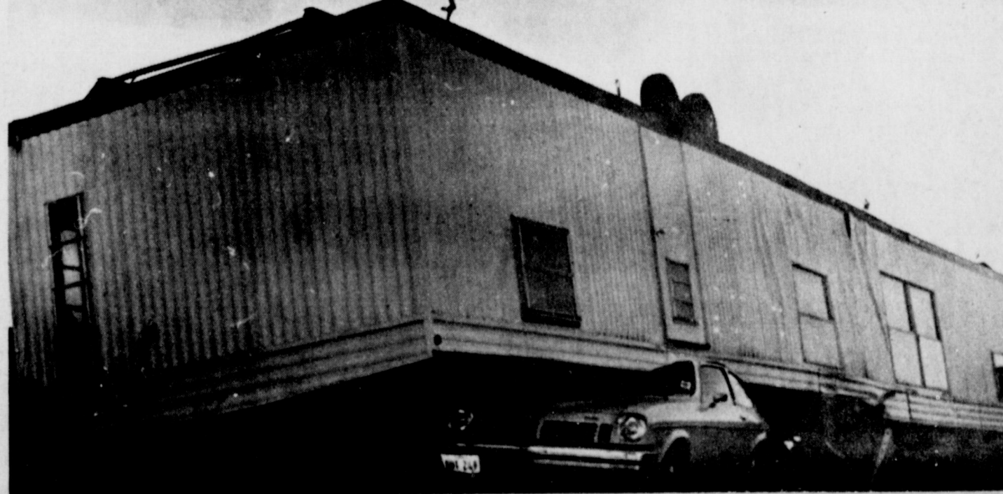
TRAILER LANDS ON CAR . . . The terrific wind storm in the Muleshoe area Saturday, picked up this trailer home belonging to Gerald Haddon and dumped it upside down on top of a car belonging to Rodney Turnbow. The trailer was moved several feet from its foundation before coming to rest on the car. Considerable damage was done to the trailer as well as its contents and the Turnbow vehicle.
