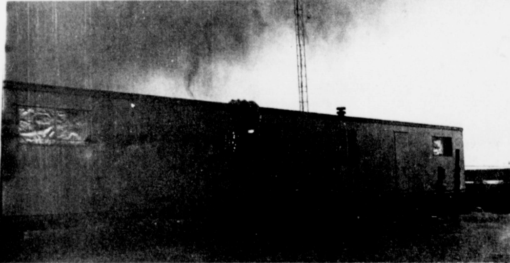
WIND DAMAGED . . . this trailer home in the Ranch House Trailer Park located on West American Blvd. in Muleshoe during Saturday's wind storm. The curtains are shown blowing outside and one can see what appears to be a small funnel cloud in the center of the picture.
