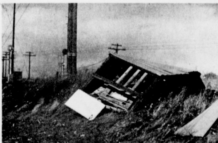
SMALL SHED . . . belonging to Tom Flowers on U.S. 84 was picked up by high winds Saturday, carried across the highway and dumped in the bar ditch.
