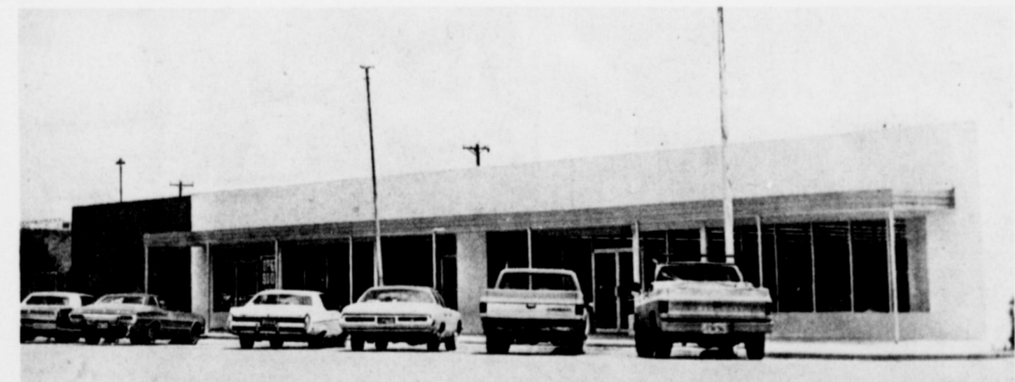
NEARING COMPLETION . . . Construction on the new Anthony's store for Muleshoe is nearing completion, with the opening date before the end of this month. Lindal Murray, manager of the
