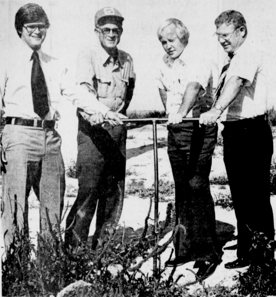
TURNING THE WATER ON... Monday morning, a long-awaited event took place for the city of Muleshoe. Quietly and without fanfare, city officials turned the water on to fill the new 1,000,000 gallon water tank in the background. The elevated tank was turned on by from left, Jack Eades, assistant city administrator; L.M. Bell, water superintendent; Dave Marr, city manager; and Kenneth Henry, Muleshoe Mayor.
