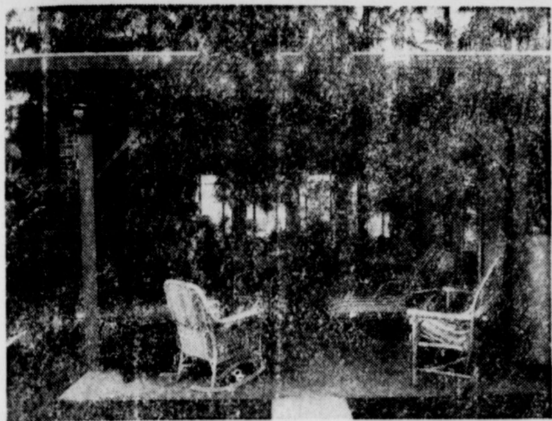
GARDEN SHELTER. This rustic garden shelter was built by the owner with nothing more than framing members, six panels of exterior fir plywood and a set of old French doors salvaged from an earlier remodeling job. Shelter has practically doubled the time the family can spend in outdoor living.
