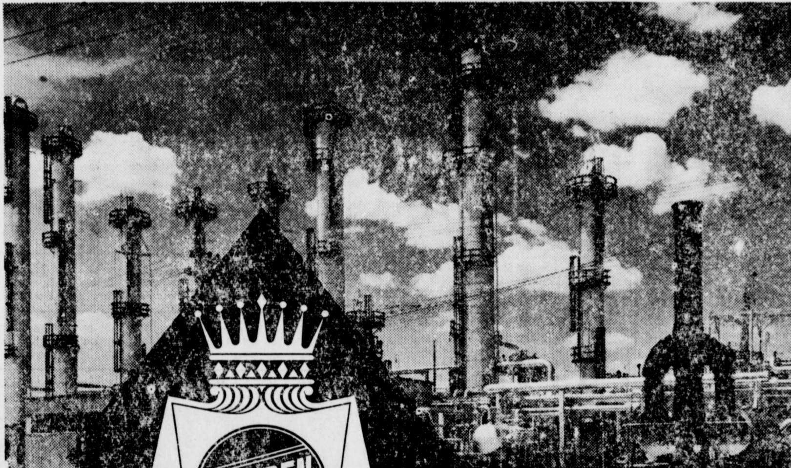
PARTIAL VIEW OF COSDEN'S MULTI-MILLION DOLLAR REFORMING UNIT
