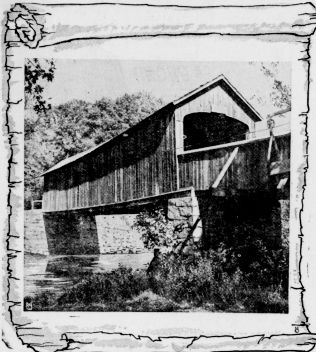
HAVEN OF SAFETY IN A SUDDEN STORM
