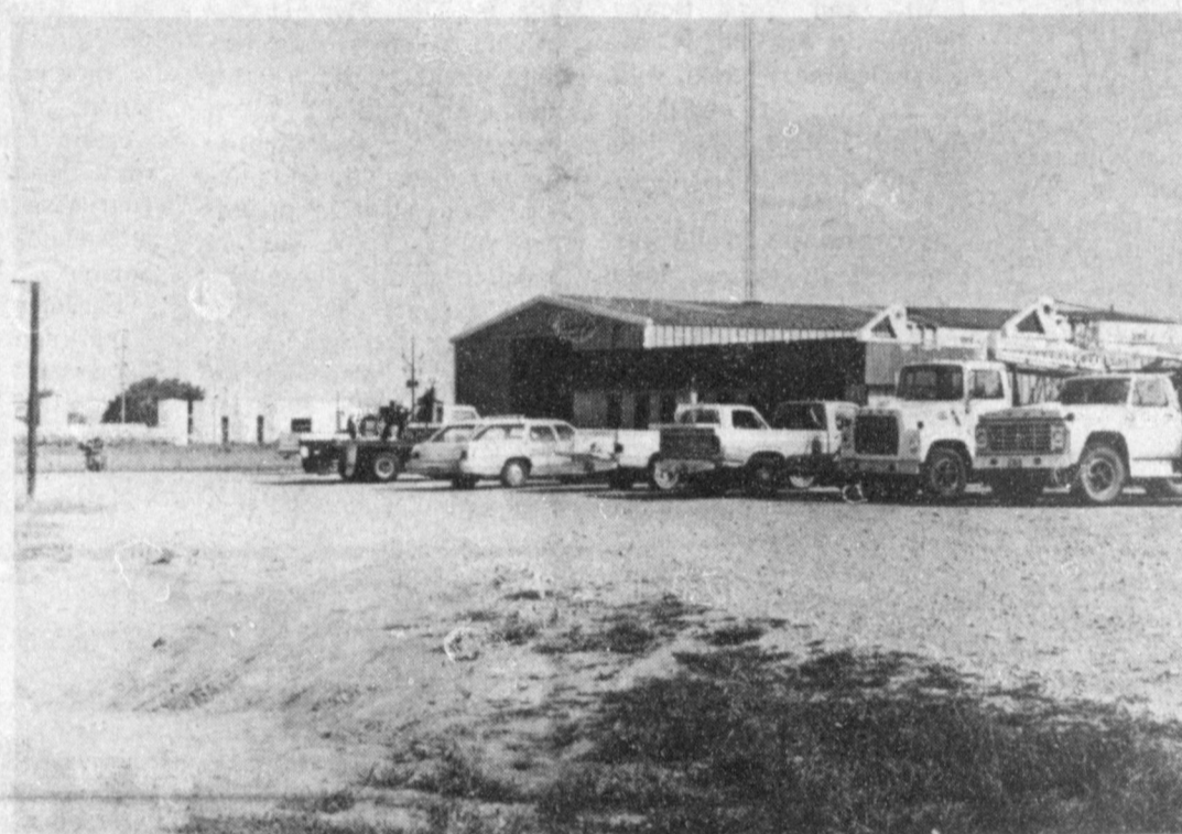
Irrigation Pumps & Power
