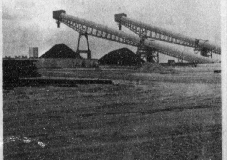
COAL STOCKPILE... The Tolk Plant now has reached and surpassed its 90 day stockpile of coal. (290 thousand tons). This amount will allow the plant to run 90 days in the event of a strike or of the coal being undeliverable. When the second unit is completed about 500 thousand tons will be necessary to stockpile for the 90 days ahead.
