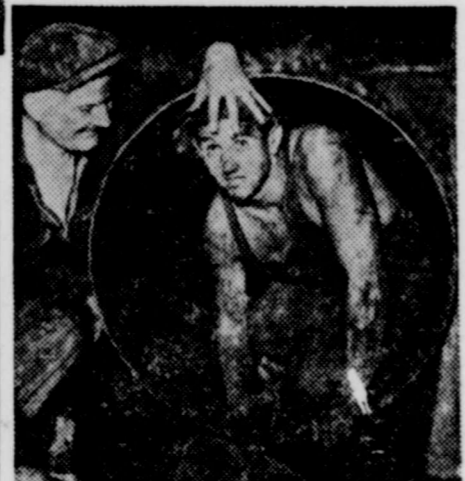
HOLED THRU—The Midtown Hudson Tunnel which, when completed, will link New York City with Weehawken, N. J., was "holed thru" recently when the 400-ton shield which works from the Jersey side have steadily pushed forward for 18 months bumped into the New York shield.
