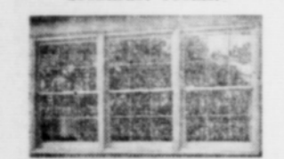
A multiple bank of double hung windows, often used at the end of the living room.
