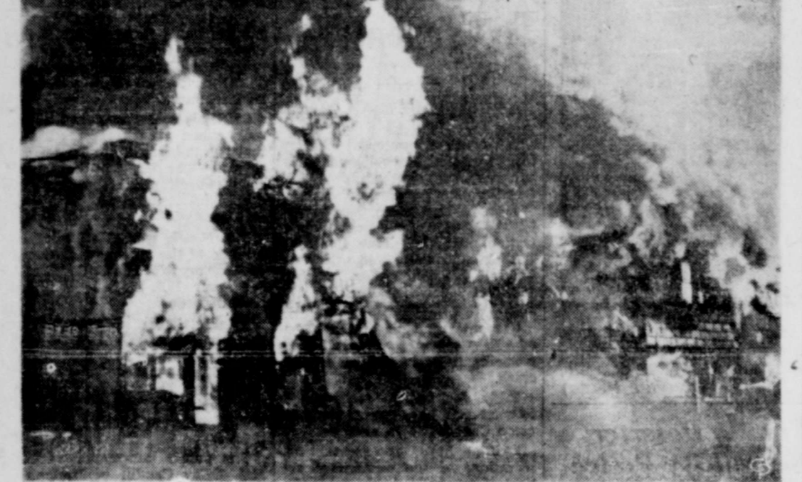
FLAMES LEAP HIGH from eight-family Fairbanks, Alaska, apartment where 14 died after U. S. Air Force Thunderjet crashed into structure shortly after taking off. (International)
