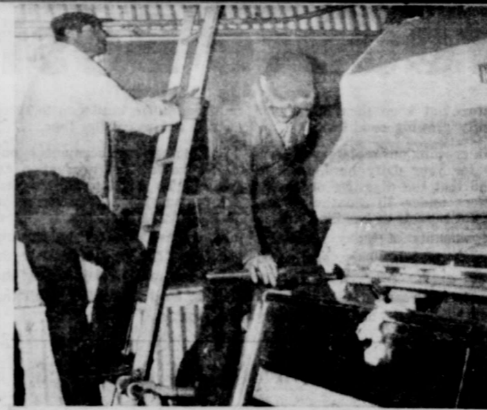
REPAIRMEN get at a trouble.
