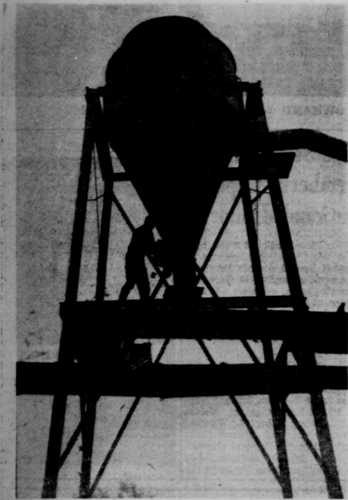
CLEANING a trash collector at the gin.
