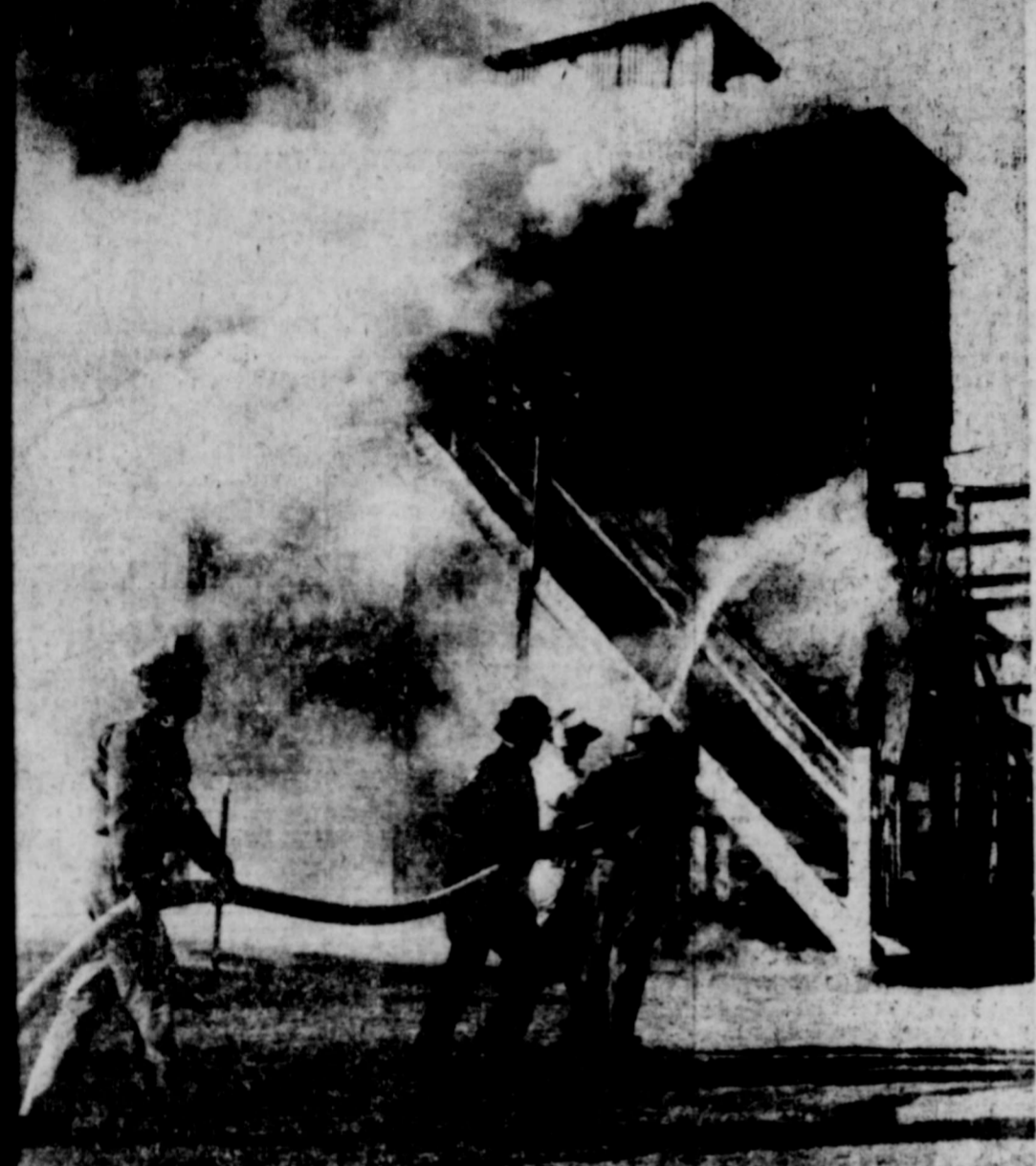
FIRE DESTROYS press box structure at Morris Field in an 8:37 a. m. blaze today. The fire started in a shed beneath the press box and swept through the structure before men could get water to it. (Advocate Photo)
