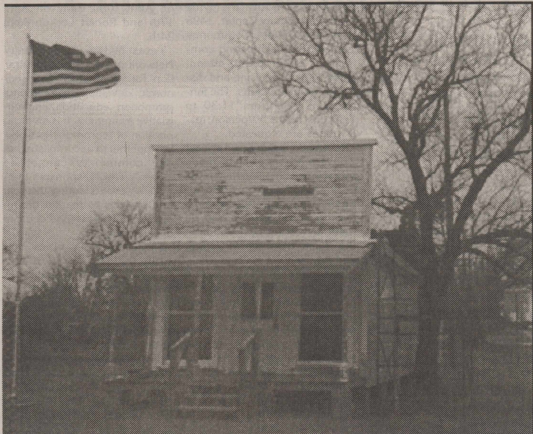
Restoring a Part of Cottonwood History — The old Cottonwood Post Office is ready for a fresh coat of paint. The Cottonwood Historical Association Board Members has been working on the building.
