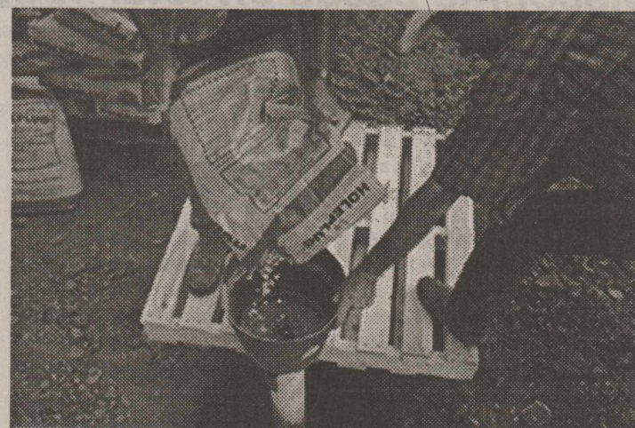
LANDOWNER PROTECTS AQUIFER AND WATER QUALITY BY SEALING ABANDONED WATER WELL
