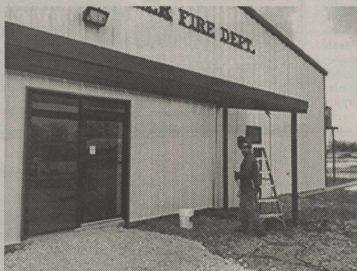
Josh Loftis working on the front entrance of new firehouse
