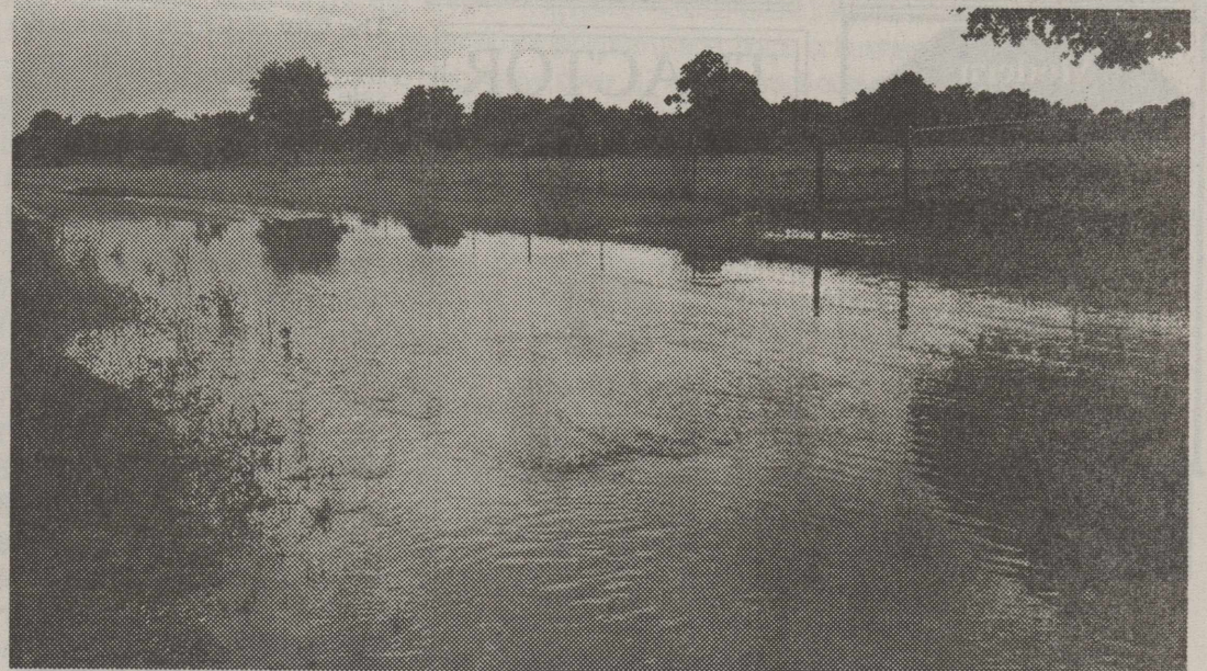
Flooding on one of the Country Roads in Cottonwood
