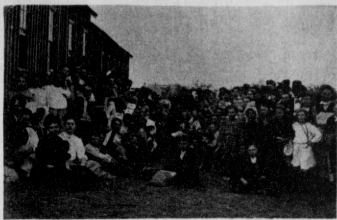
ROTAN'S FIRST SCHOOL: White Flat was a 3-section wooden building, 1907-1909.
