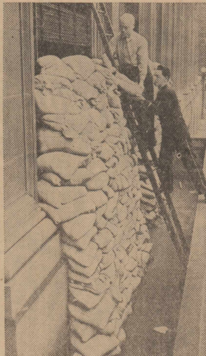
Completing the job of placing sandbags outside the office windows of Hotel Bossert in Brooklyn. The barriers were installed so the hotel organization could keep functioning in case of an air raid.
