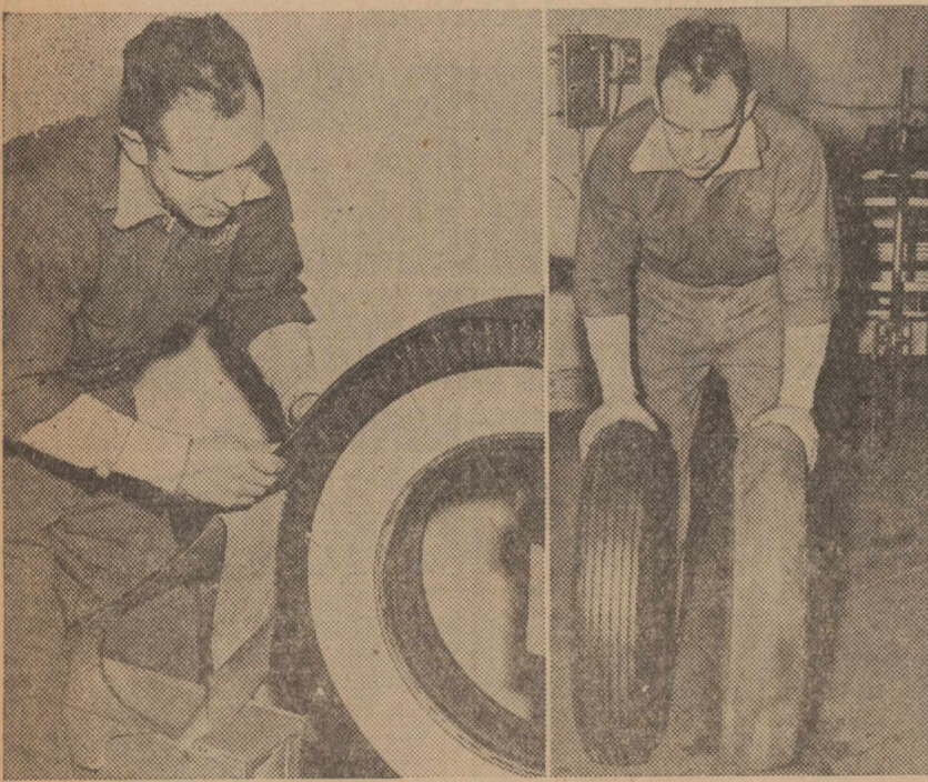
We will all have to do without new automobile tires for the present. Next best thing is a retreading job on your old ones, if they are too smooth for safety. At left you see a re-treading operation in progress. A "camel back," or new rubber top, is vulcanized to the old casing to give a new gripping tread. At the right is shown how a worn-out tire compares with one that has just been given a face lift, or a new tread. The recapped tire is at left; the old "smoothy" beside it.
