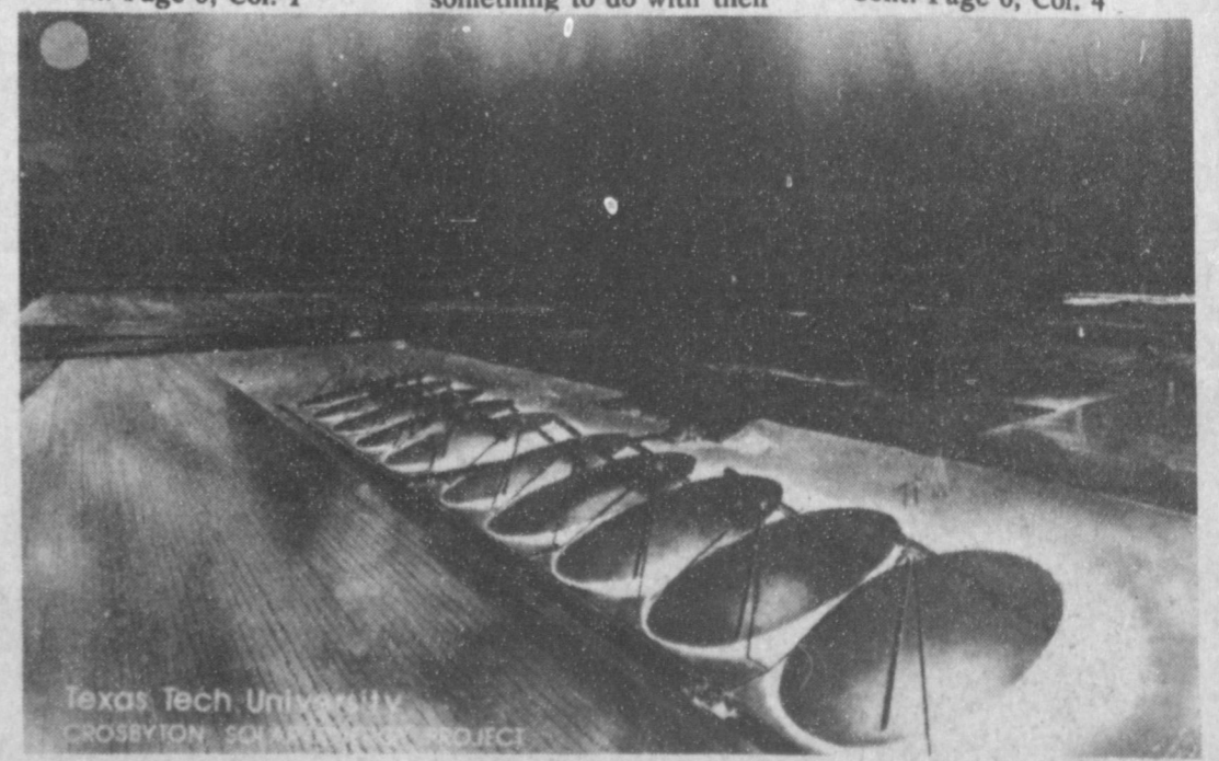
SOLAR POWER PROJECT. The Crosbyton Solar Power Project has been operating for over two years, successfully. Pictured are ten two hundred foot diameter glass bowls which power the unit. Over four hundred thirty thousand square feet of mirror space is in these bowls and the temperature reaches up to eighteen hundred degrees at times. Rotary guest Col. Travis Simpson of Texas Tech presented a program on the operation and working of the solar power unit.
