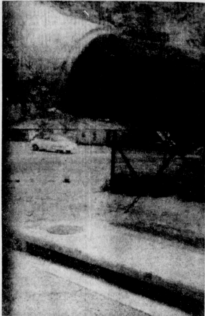
NO MORE FLOODING — Downtown flooding of streets during heavy rains has been eliminated now with the completion of new storm sewers, part of a big bond-financed project to improve sewer system in Muleshoe. Top picture shows the storm sewer drainage at extreme southeastern edge of town. Bottom picture is a storm sewer at W. Ave. B and Fir St.
