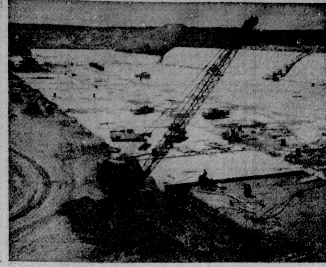
SPILLWAY NEAR COMPLETION
