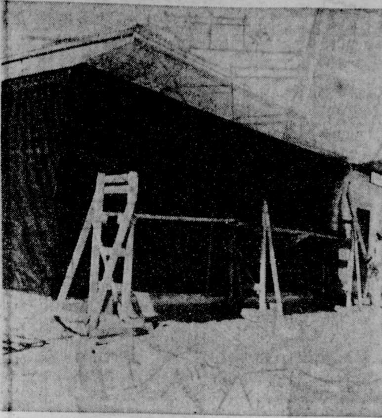
NEW BUILDING — Construction is now underway on a new building picture above being erected by businessman W. D. "Bill" Moore. The new structure is located across the street south of the Courthouse.
