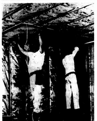
EXTRA ROOMS, EXTRA HEATING - Home expansion is a popular solution to the family living crunch, but added rooms mean additional heating needs and may tax existing heating systems. Radiant electric heat from special ceiling panels offers a very practical way to expand the present home heating system
