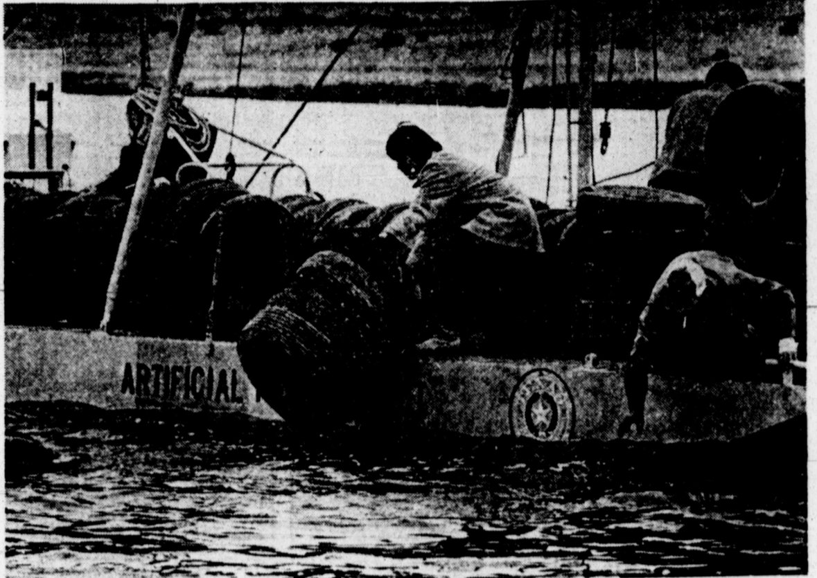
RUBBER REEF —The Texas Parks and Wildlife Department has found a way to recycle old automobile tires—make reefs out of them. Above, three Parks and Wildlife employees with the department's Artificial Reef Project hurl the tires into the water of Canyon Lakes No. 1. From left are Kirby Gholson, Robert Castillo and Domingo Canales who concluded their bosses could have found better weather than that on Tuesday for work on the project. The artificial reefs are formed when the tires sink to the bottom of the lake and allow the formation of underwater growth. (Staff Photo by Holly Kuper)
