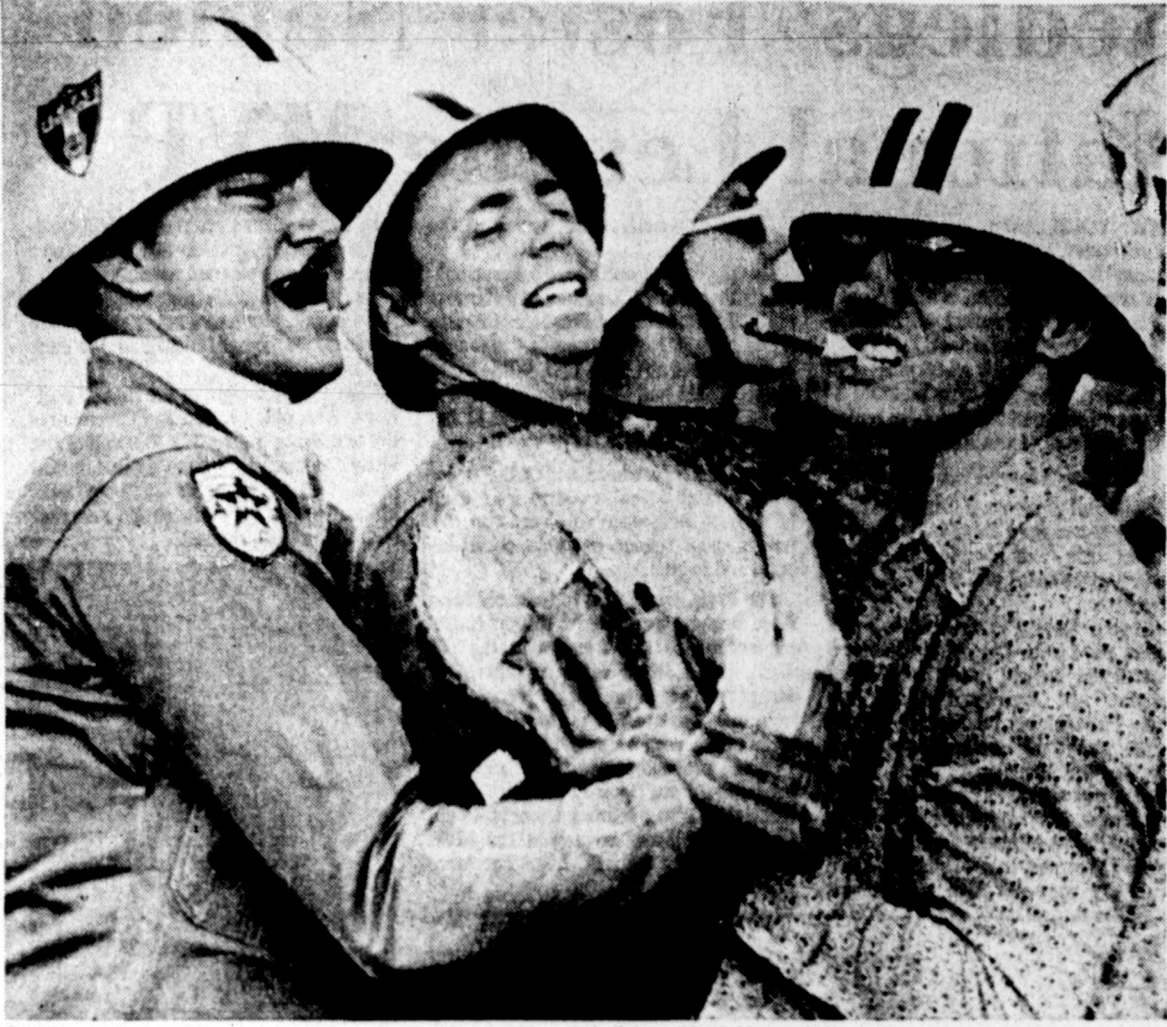
BONFIRE BUILDERS —Texas Aggies this week have begun construction of their annual bonfire, scheduled to be ignited Friday, Nov. 25, before the Texas A&M-Texas football game. The two, chopping down on cigars as they lift logs onto the pile, are Mitch Namendorf and Bruce Cummings, left and right, of the Aggie Corps of Cadets. The 80-foot centerpiece went up Monday and the Aggies hope to have a stack of lumber almost as tall as the centerpiece. (AP Laserphoto)
