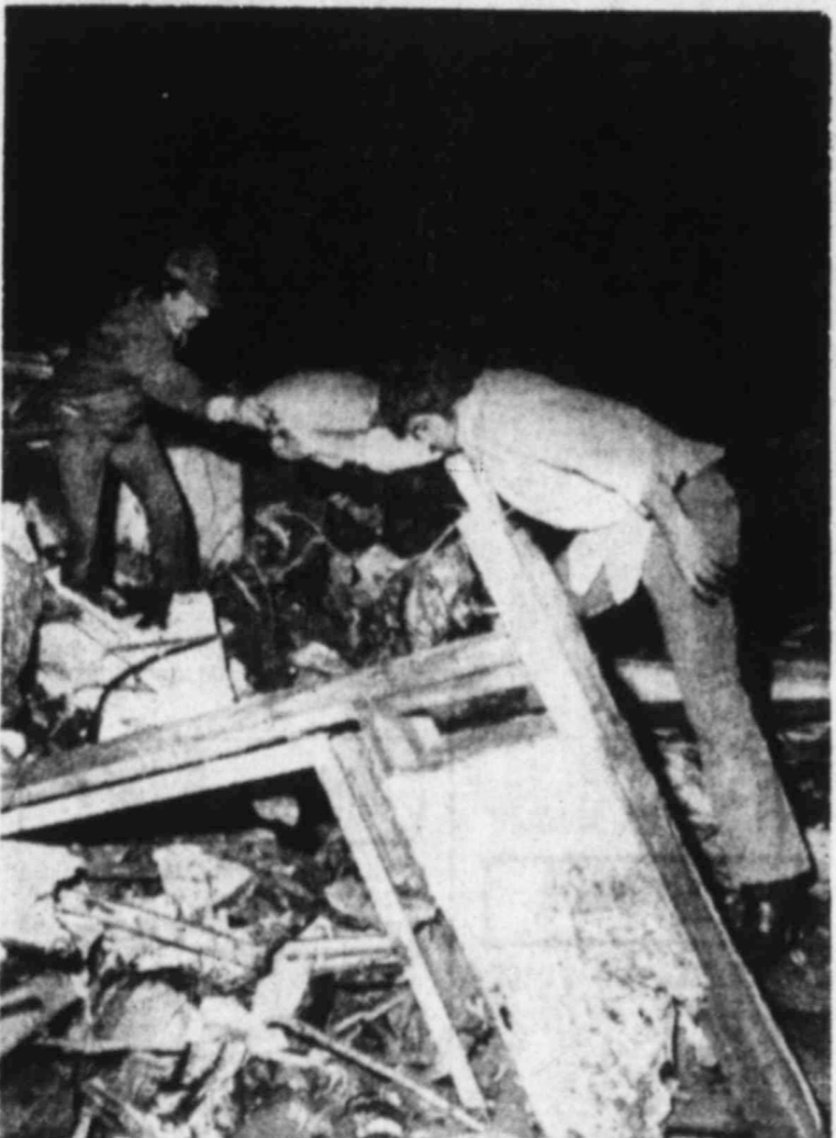
TORNADO'S FURY — Two men search the remains of a building in Wichita Falls Tuesday night for survivors of the tornado that swept through the city causing death and destruction. (AP Laserphoto)
