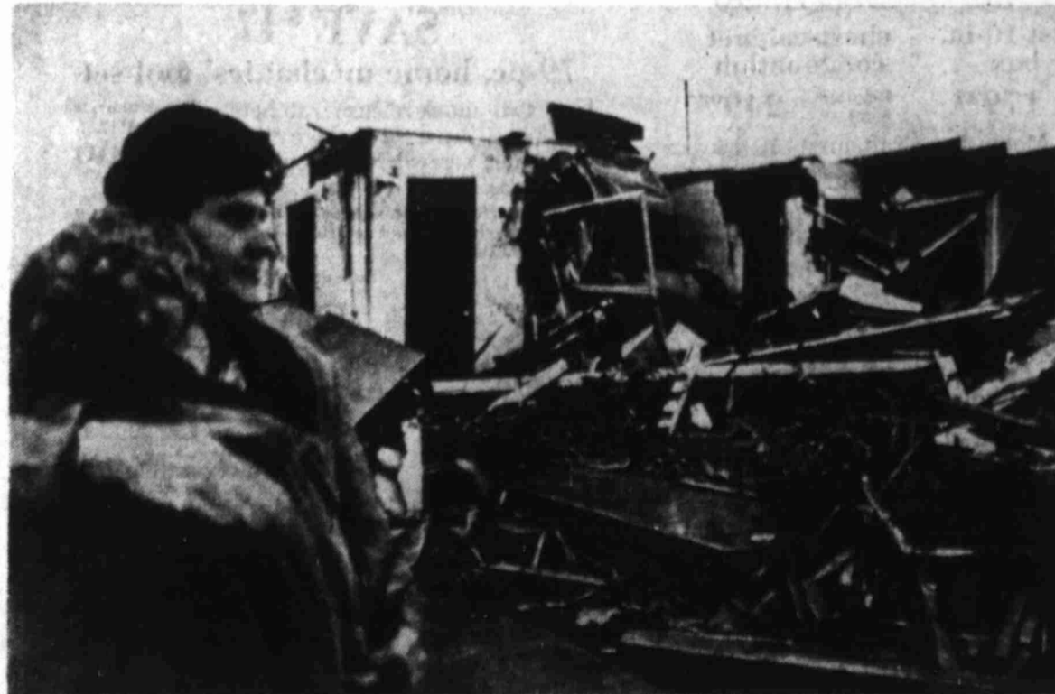
DAMAGED HOMES — An unidentified family surveys the damage to their home after a tornado wrecked portions of Wichita Falls Tuesday afternoon. An automobile, in center of photo, was tossed on top of the rubble. (AP Laserphoto)
