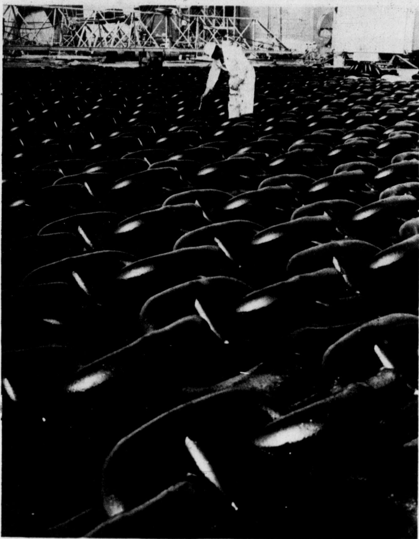
This painter at Tenneco Inc.'s Newport News Shipbuilding subsidiary in Virginia puts the finishing touches on more than 1,400 links of anchor chain for an ultra-large crude carrier (1,187 feet long, 390,000 deadweight-tons), the largest ship ever built in the Western Hemisphere.
